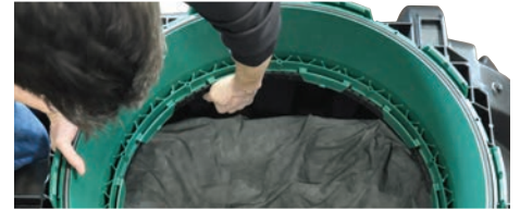
Engage one set of tabs into proper position.
