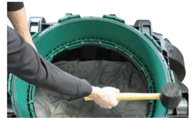
Use mallet to engage the rest of the tabs.
